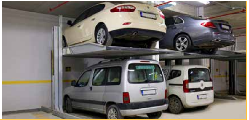
İstanbul, Beşiktaş, Etiler, Lale Apartment Ofton Construction Co. Mechanical Parking System
