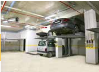
İstanbul, Beşiktaş, Etiler, Lale Apartment Ofton Construction Co. Mechanical Parking System
