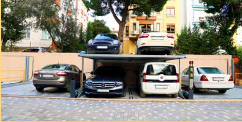
İstanbul, Maltepe, Denizkent Apartment DKD Construction Co. Mechanical Parking System
